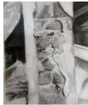
Plate X: Preliminary drawing of an exposed block work as a result of cracks on the wall,
